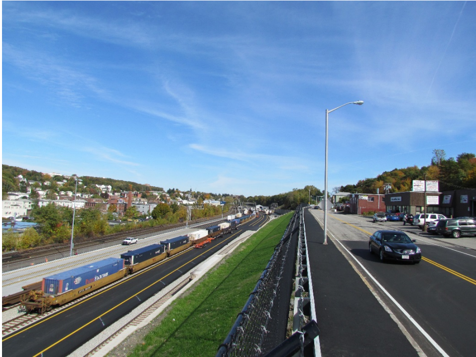
Roadway improvement above
