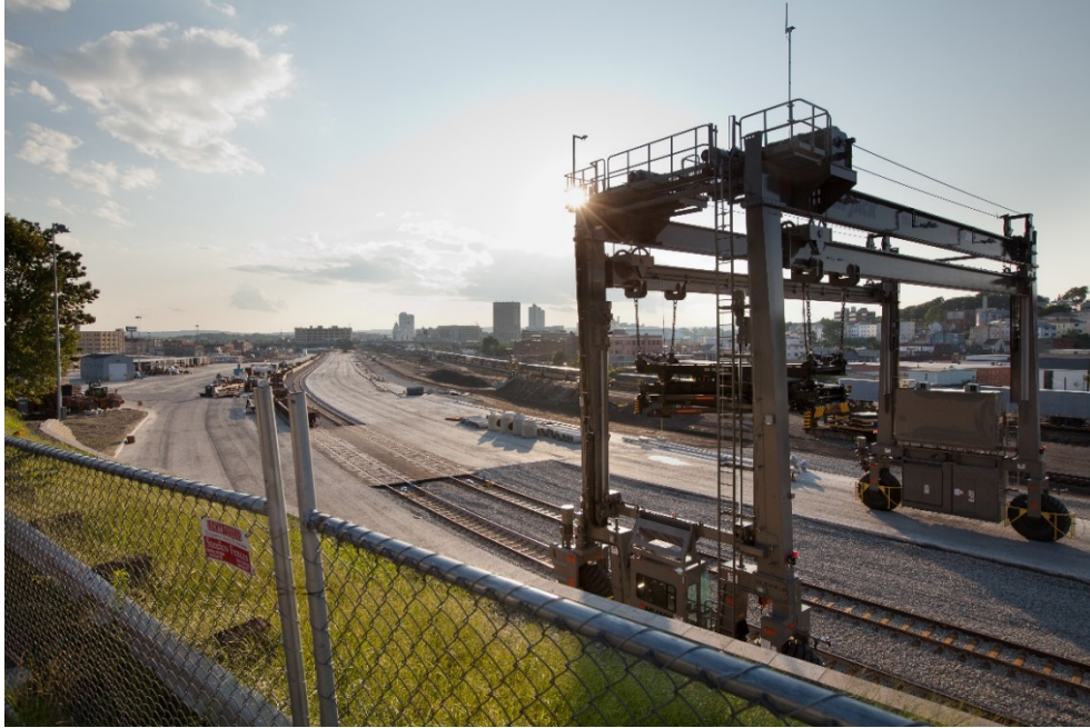
Railway expansion completed
