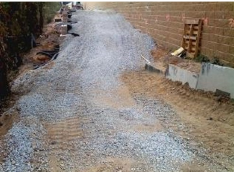
Start of the new buttress wall and temporary shoring
