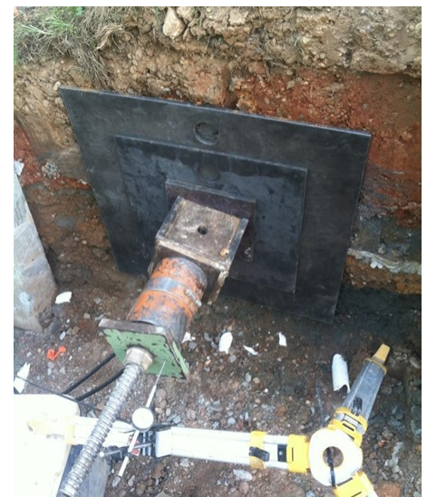
Nail Testing & Lock-off
