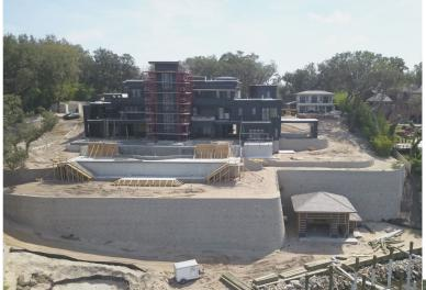
Compared to alternative designs and retaining wall types (big block walls, soil nailing, poured -in-place concrete walls), the ERS-designed segmental retaining wall (SRW) solution achieved cost savings of over 60%.
