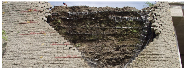
Figure 6 Wall Failure Due to Improper Quality Control
