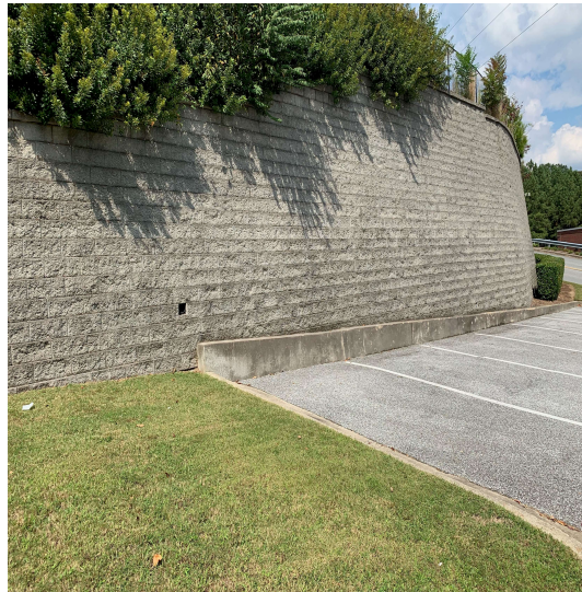
Figure 5 Bottom of Retaining Wall at Wrong Elevation for Standard Curb
