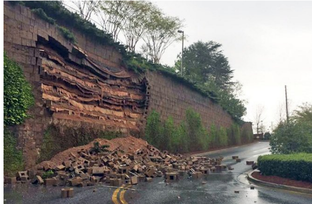
Figure 1 Wall Failure Due to Unsuitable Soil
