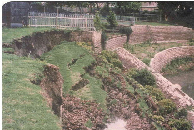
Figure 2 Global Stability Wall Failure
