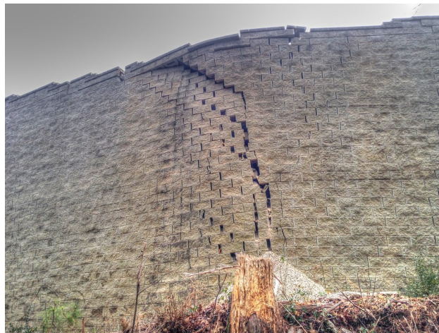
Figure 3 Wall Settlement Due to Unsuitable Foundation Soils
