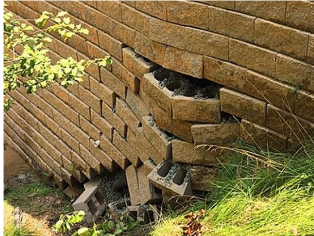
Figure 7 Bottom of Wall Erosion Due to Poor Surface Water Management
