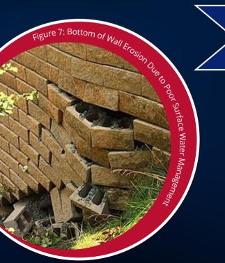
If the surface water is not directed to an alternate location, there is a high probability that a significant rainfall event will cause severe erosion and possible failure of the earth retention structures.
