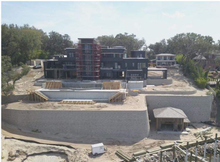
Working closely with ACP, a large retaining wall installer in Florida, ERS was able to coordinate the stamped engineering, site supervision, and wall installation with the architect and general contractor. The result is a spectacular home, placed atop a fully geogrid-stabilized soil mass, with all required factors of safety. **The result: an architecturally beautiful solution to a tough site, and a satisfied owner.**
