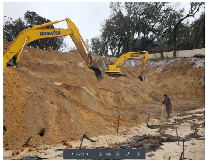
The initial retaining wall analysis was performed by a national retaining wall company. Their design did not include a more rigorous global stability analysis which considers potential deep-seated, rotational failure surfaces outside of the traditional “reinforced soil zone”.
