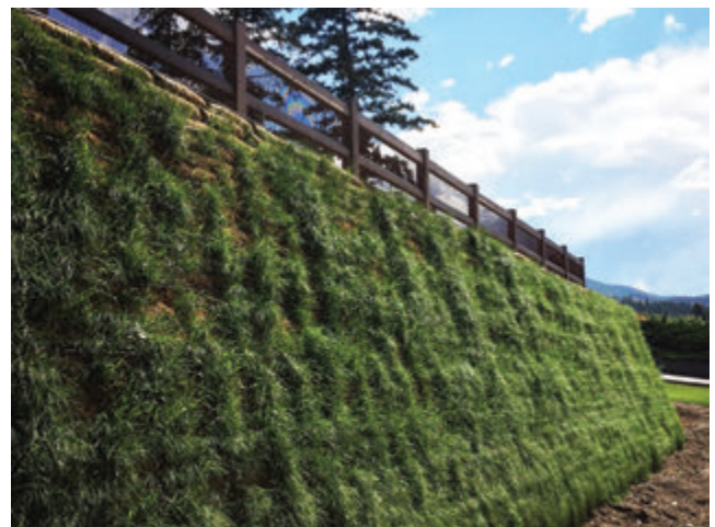
5m (16ft) tall landscape retaining wall
